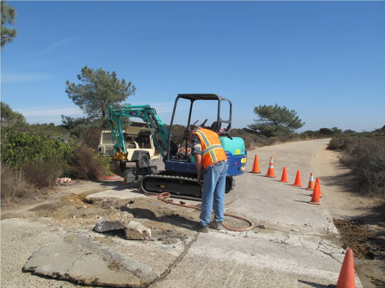
FIGURE 17. TORREY PINES PARK ROAD UNDER REPAIR, NOVEMBER 2011.
